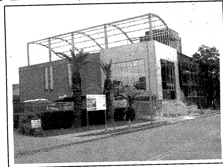
Additions to the Chabad Lubavitch Center are already underway.
